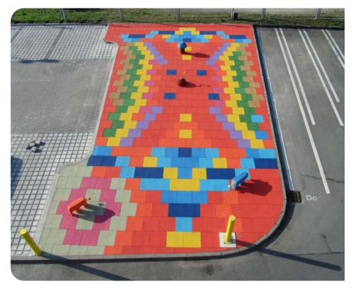
loosely poured impact protection such as sand or bark mulch, which has to be regularly raked, redistributed and, if necessary, filled up, the impact protection panels constantly retain their original thickness and thus the required impact protection properties. Contamination or dangerous objects such as shards are immediately visible and can be removed without difficulty.
